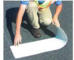
Fig. 2 Position PreMark® material according to diagram provided
