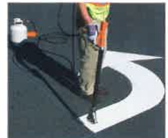
Fig. 3 Heat PreMark® material according to instructions.
